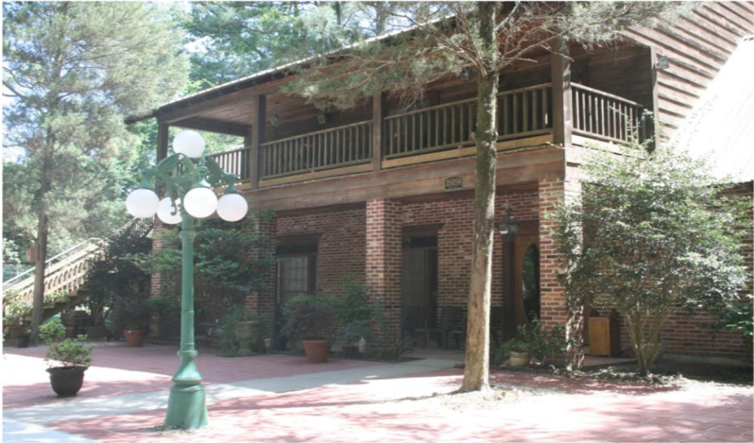
Lodge (course rooms, male quarters, and offices)
